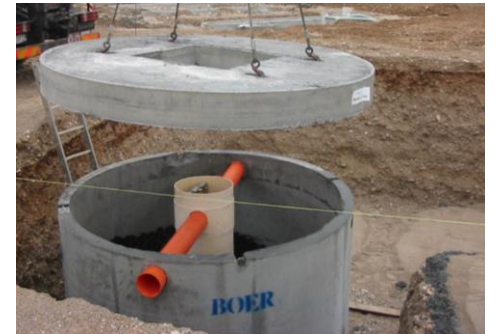
Water treatment and purification
